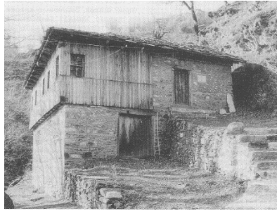
Figure 4: Monolithic expression by stone and timber framing – the house of Gjorgji Pulevski in Galichnik – image from Brezoski (1993)
