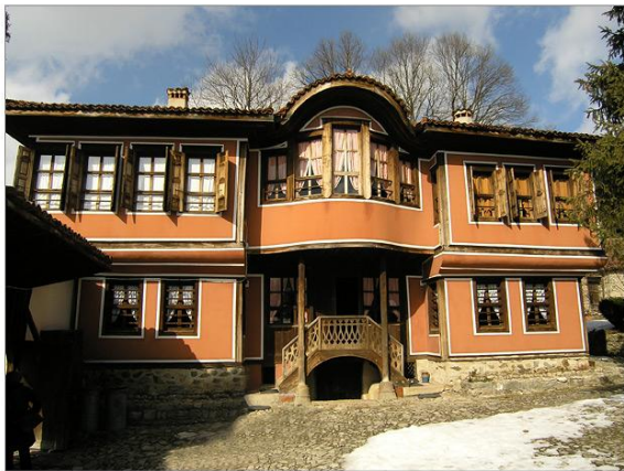
Fig. 7. Kableschkov House in Koprivshhtiza, Yard Façade.
