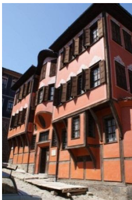
Fig. 3. Dimitar Georgiadi House in Plovdiv, Street Façade.
