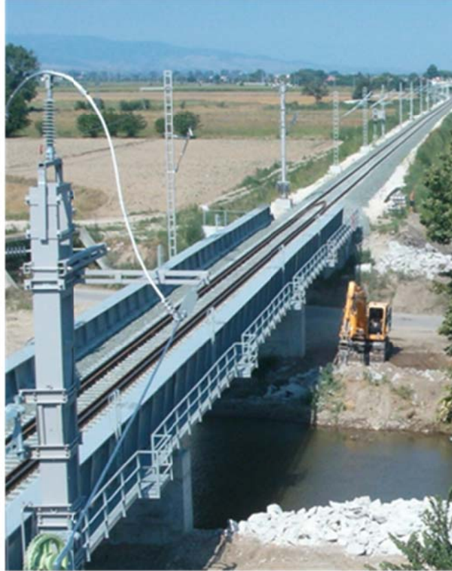
Figure 3: Bridge over Chaya river
