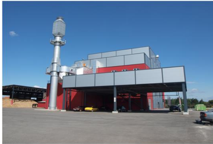
Figure 2: Municipal heating plant using wood chips, Topolčany, Slovakia
