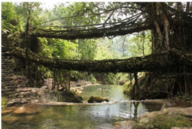
Image 5: Double Decker Living Root Bridge
